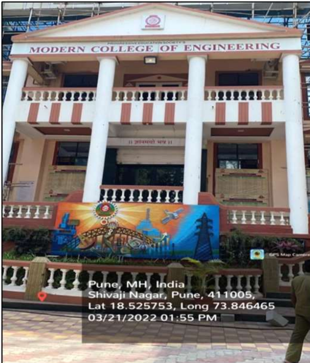
Front View of Main Building
